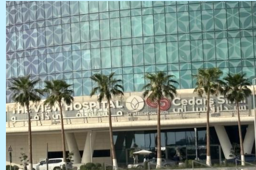
Main Entrance Gate
